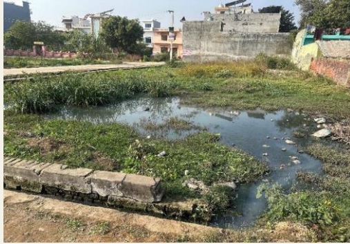
Drain outfall in open land in ward 6
