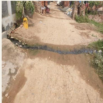
Kachha drain crossing road in ward 7
