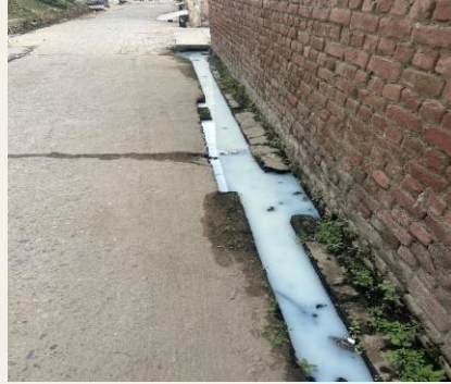
Drain carrying chemicals in ward 6
