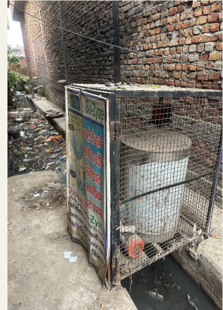
Defunct bioremediation system in ward 13
