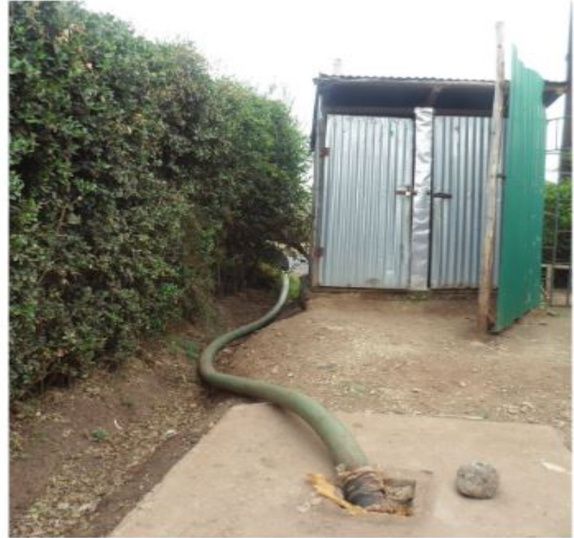
Figure 2: Septic tank being emptied by a vacuum truck ©GIZ/Doreen Mbalo
