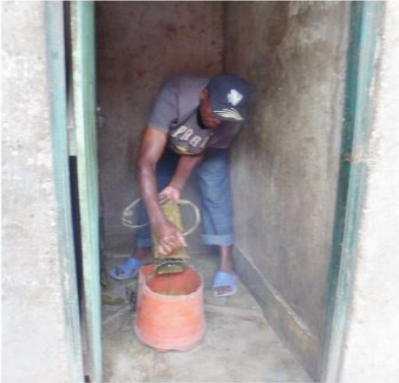
Figure 1: Manual emptier emptying a pit latrine with a bucket ©GIZ/Doreen Mbalo
