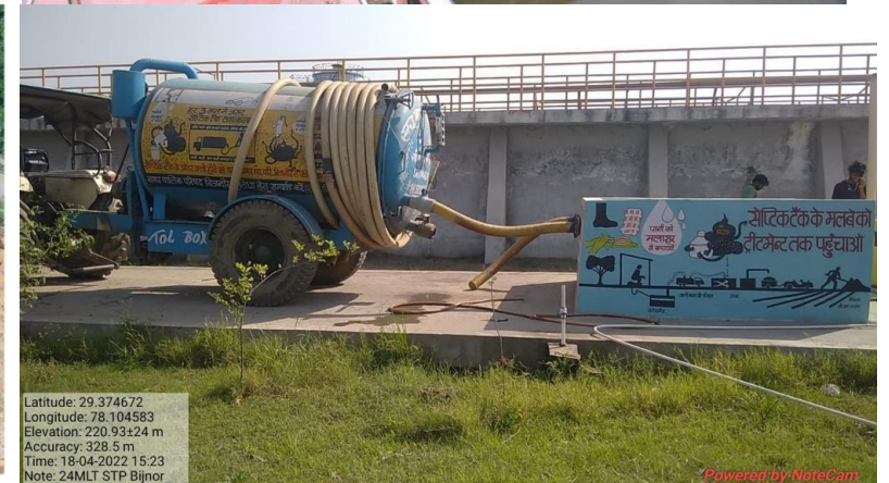
Co-treatment plant – Bijnor, UP
