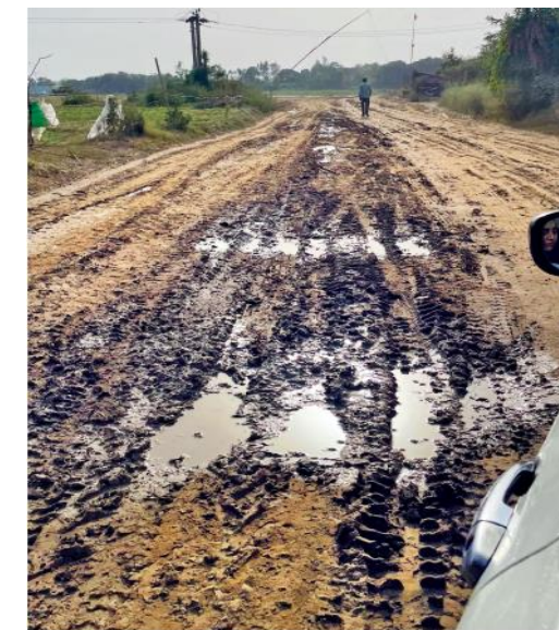
Improper approach road to FSTP in Pilibhit
