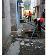
Mechanical emptying of faecal sludge by overnment operated tractor mounted
