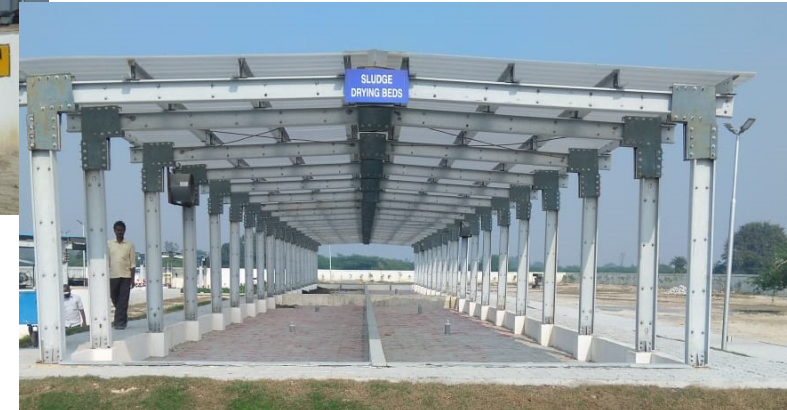
Drying beds covered by polycarbonate sheets
