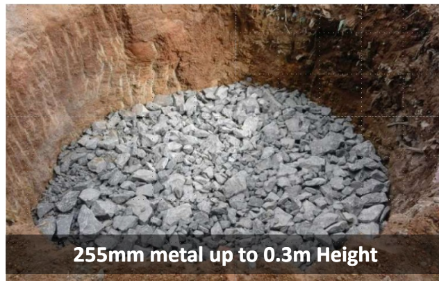
EARTH WORK – 4m Diameter and 1.8m Depth
