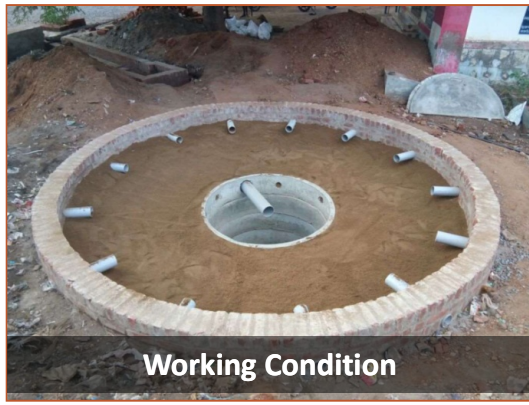
EARTH WORK – 4m Diameter and 1.8m Depth
