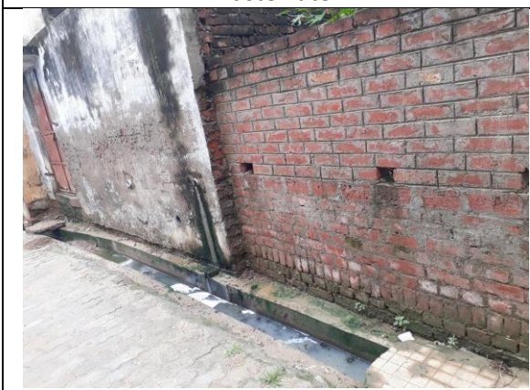
Septic Tanks constructed below toilets – Khushwaha Basti
