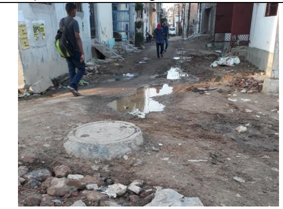
Sewer Network laid in Salori (including Narrow lanes).
