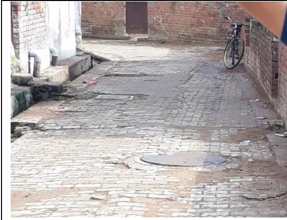
Households connected to sewerage Network in Rajapur Area near STP
