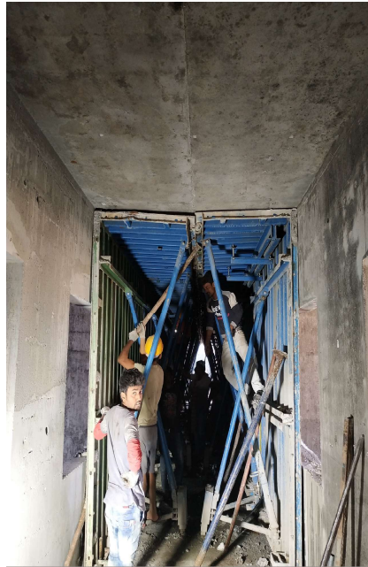
Shearwall using Tunnel formwork
