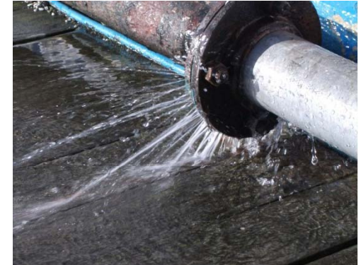
Leakage in supply lines
