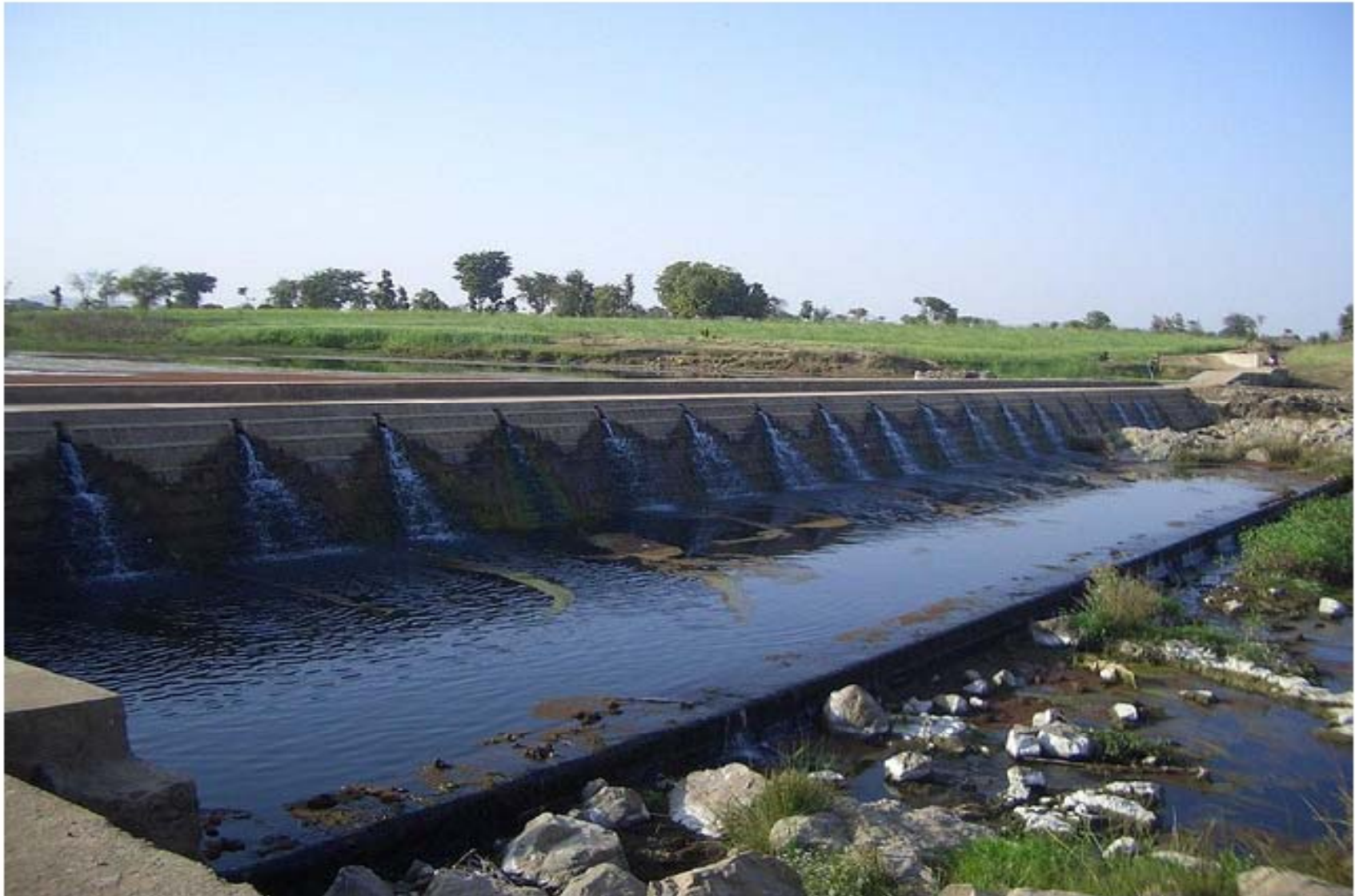
Check dam - Rajpura , UP
