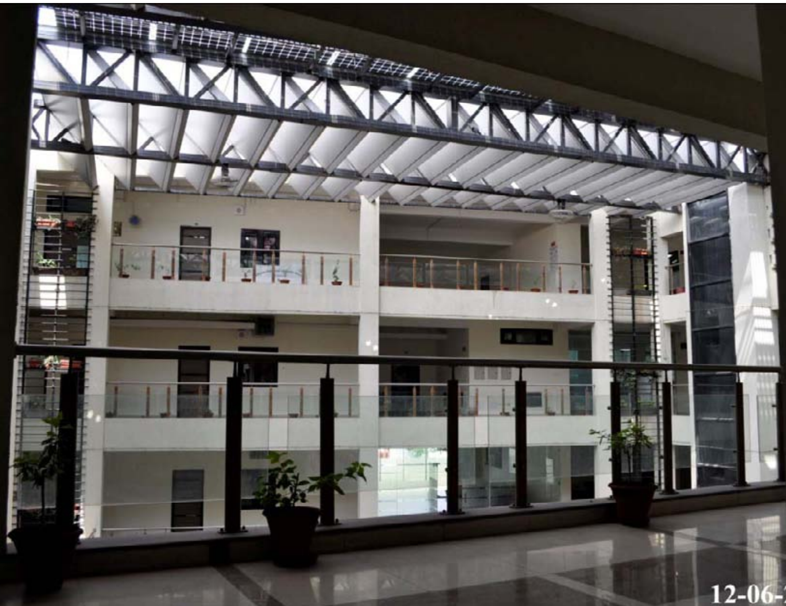
View of the louvers, B.I.P.V above the central courtyard from the first floor
