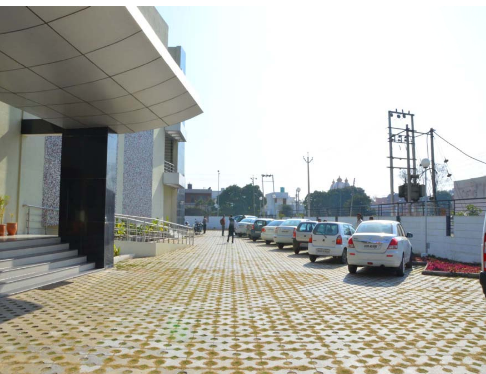
Grass pavers used as driveway floor
