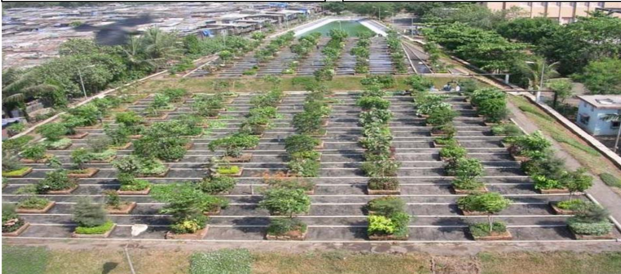
3000 KLD plant at BMC (Worli), Mumbai
