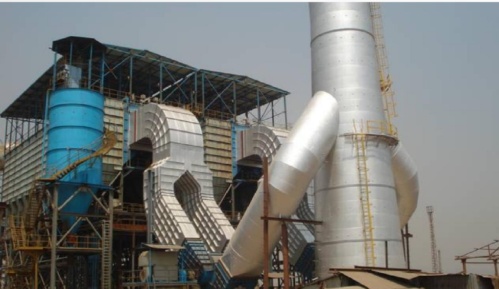
Secondary Fume Extraction(SMS-2)
