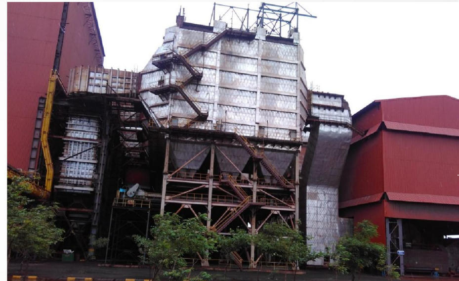
Sinter Plant-3 Process ESP
