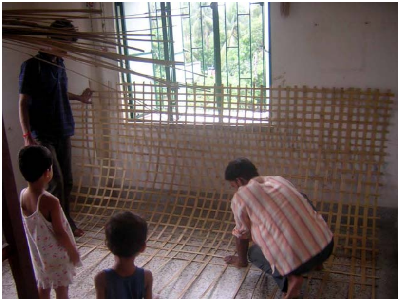
Bamboo – lime- rice husk insulating ceiling by Laurent Fournier
