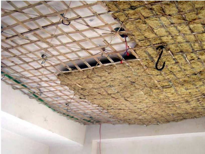
Bamboo – lime- rice husk insulating ceiling by Laurent Fournier
