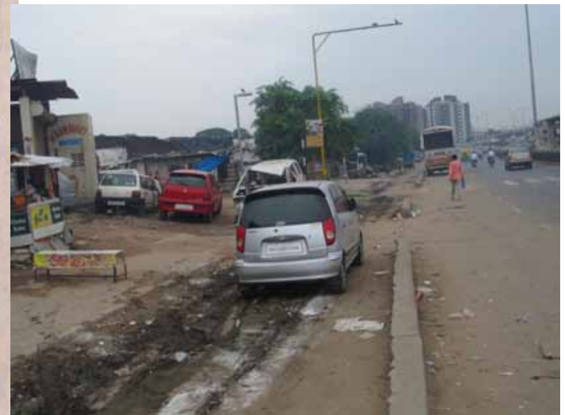
BADLY CONSTRUCTED AND IMPLEMENTED
