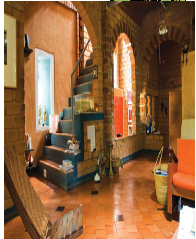
•Chitra Vishwanath's house is made of compressed stabilised earth blocks excavated from the site itself (Photo: Chitra Vishwanath)
