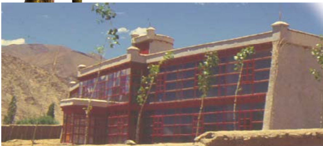
The south façade with Trombe walls caters to heating needs of the rooms
