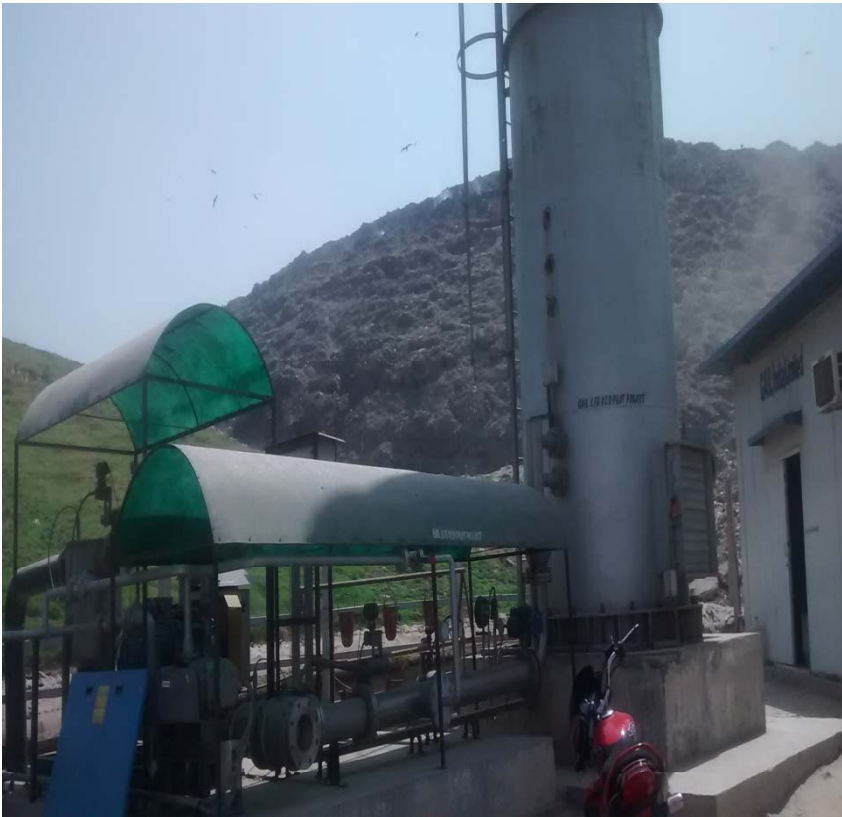
LFG scrubbing and electricity generation
