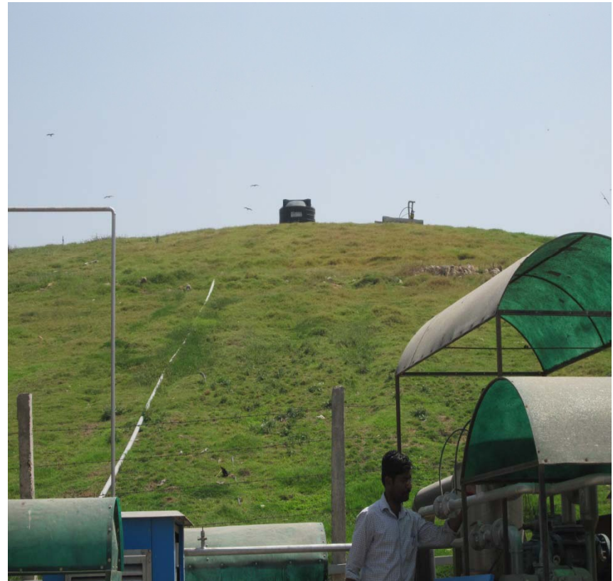
Capping and gas recovery
