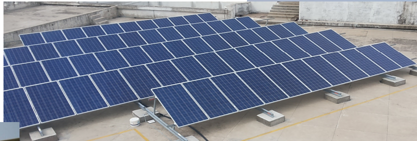
Flat RCC Roof; Ballasted
