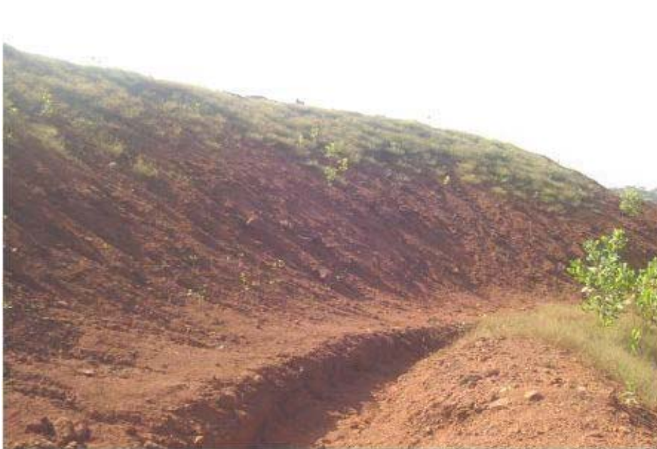
Parapet Wall Constructed Along the Toe of the Dump
