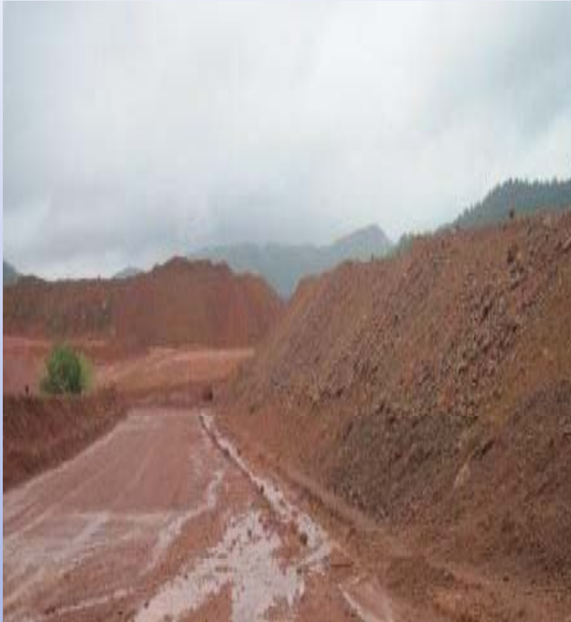
Garland Drainage Channel along the Toe of the Dump
