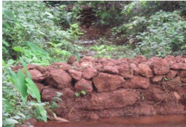
Retaining Wall at the Toe of the Dump
