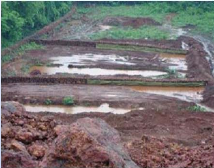
Series of silt arrestors lined with Coco filter
