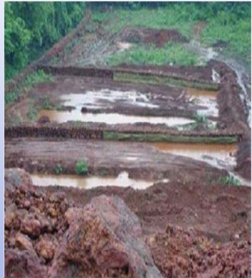
Series of silt arrestors lined with Coco filter
