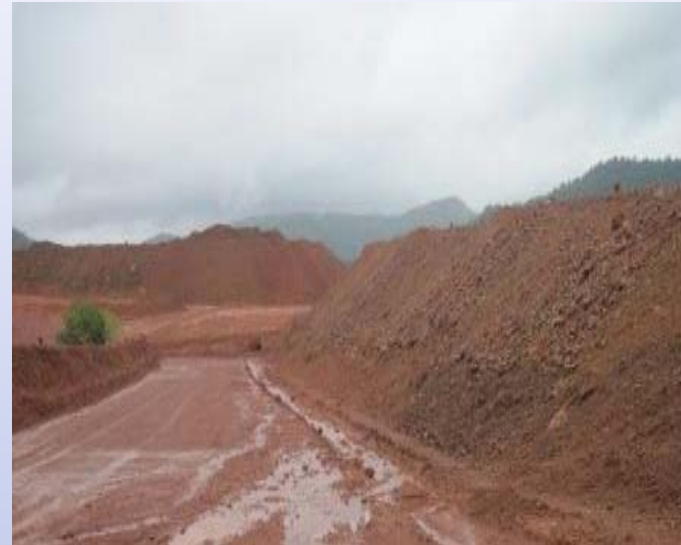
Garland Drainage Channel along the Toe of the Dump
