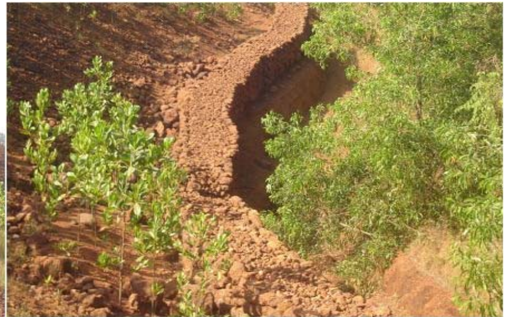
Parapet Wall Constructed Along the Toe of the Dump
