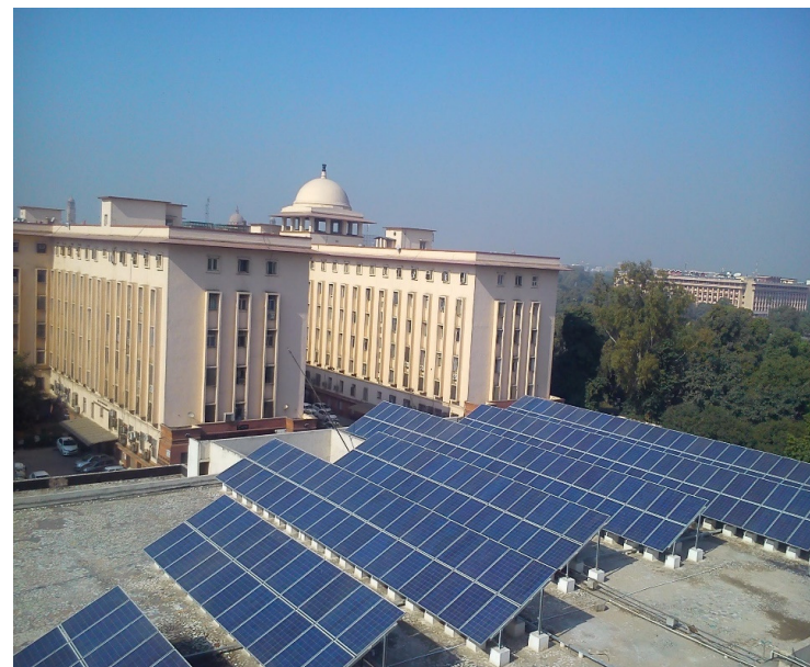
200 kWp Rooftop Grid Connected SPV Power Plant Nirman Bhawan, New Delhi
