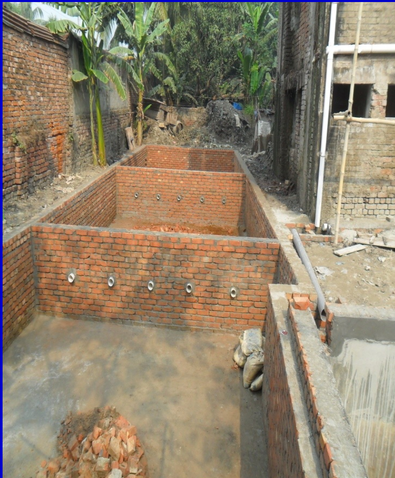
Planted Gravel Filters (aerobic treatment)
