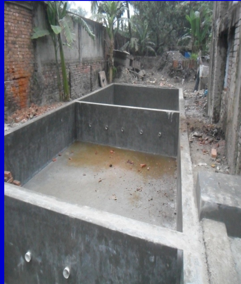
Planted Gravel Filters (aerobic treatment)
