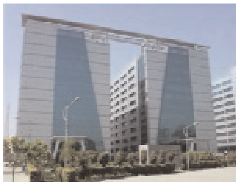
Logix Cyber Park, Noida LEED India for Core & Shell SILVER Rating
