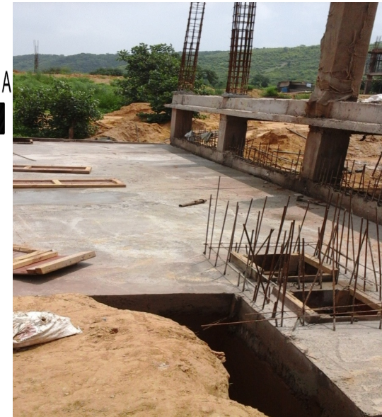
Storage Tank - Number - 2; Capacity - 100 KL (each); Use = Potable purposes
