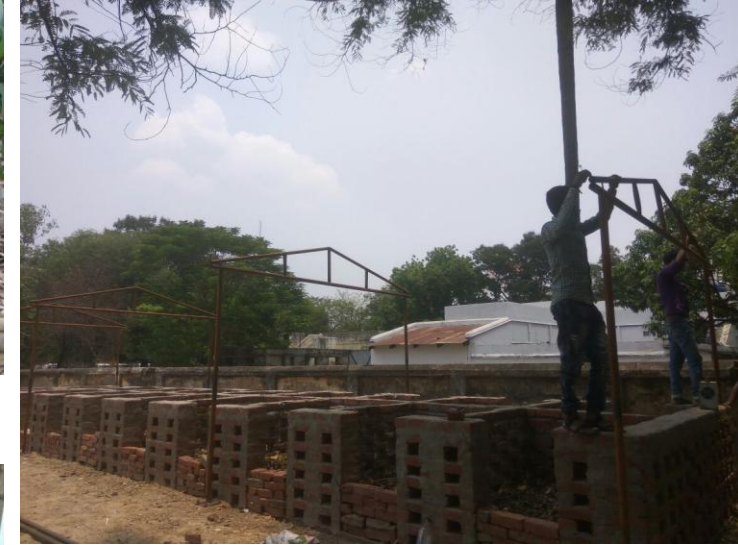
Compost pits constructed at GRDA Campus
