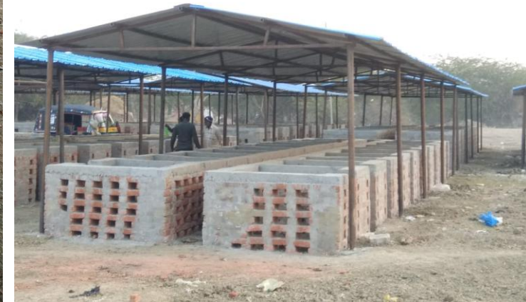
Compost pits constructed at Naili Dumping Ground
